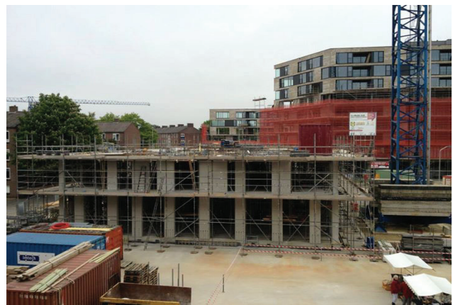
Figure 5.15 | Construction step 1 (NBU, 2013)
