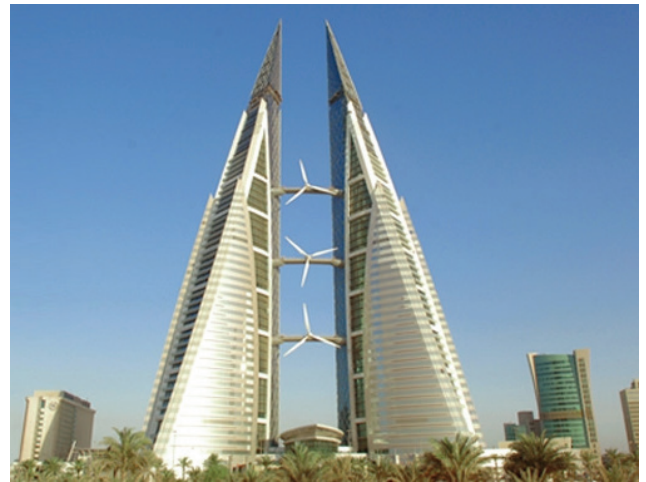
Figure 1.1 | WTC building in Bahrein (Atkins, 2007)
