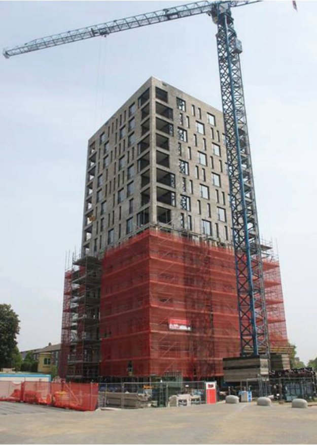
Figure 5.17 | Construction step 3 (NBU, 2014)
