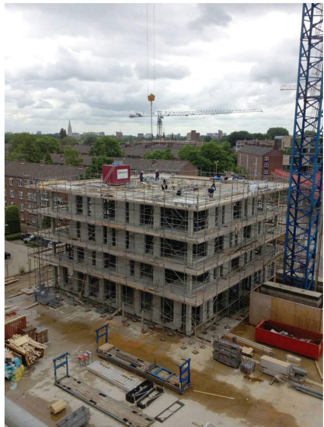
Figure 5.16 | Construction step 2 (NBU, 2013)
