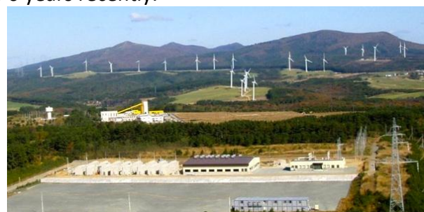
Figure 14: Sodium Sulfur (NaS) battery energy storage system (Rokasho, Aomori, Japan)
