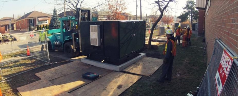
Figure 45: CES module is being installed (source: www.ecamion.com )
