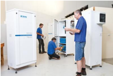
Figure 44: ZEN batteries being installed
