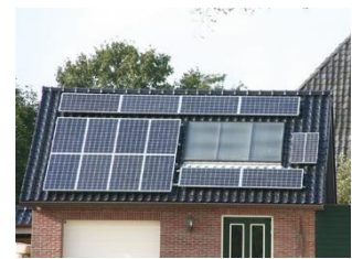
Figure 7: BAPV roof system 1
