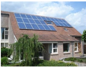
Figure 9: BAPV roof system 3
