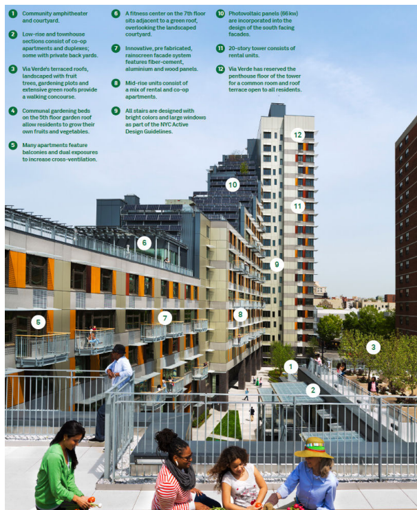
Figure 4 Via Verde Housing. From http://www.city-data.com/forum/new-york-city/286289-beyond-via-verde-green-center-south-38.html#
