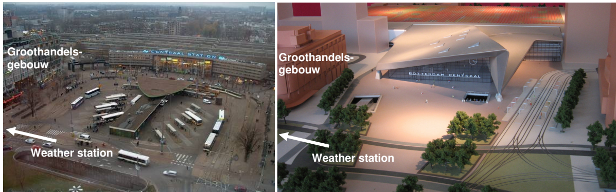
Figure 5.12: Previous train station as included in the model (left) and the current train station (right). The weather station is positioned on the southern overhang of the Groothandelsgebouw
