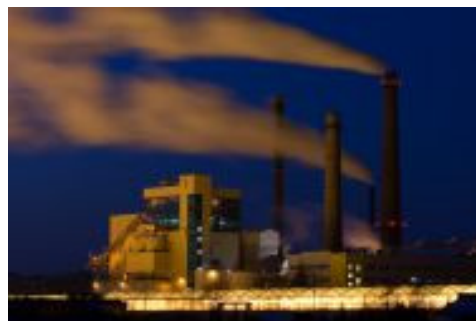
Figure 22: Biomass CHP Tartu
