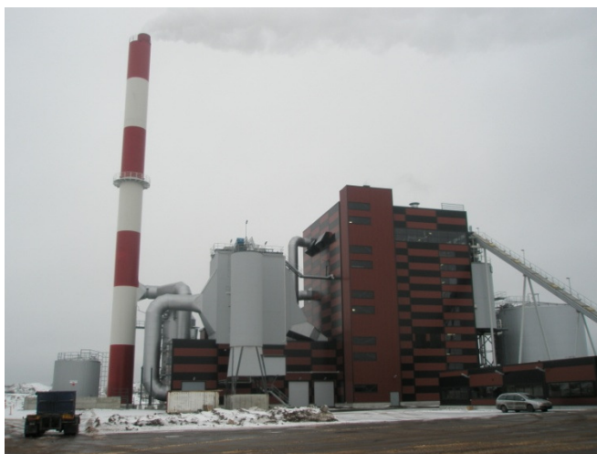
Figure 21: Vão power plant
