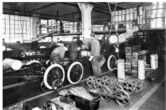
Figure 2.1 Smooth workflow through the assembly line at a Ford factory in 1913
