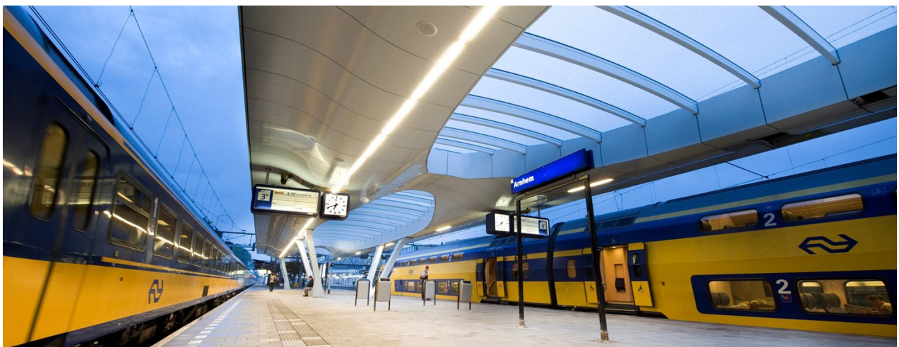
Figure 9.1 Architectural appearance of the platform roof. The two light line are running the entire platform length
