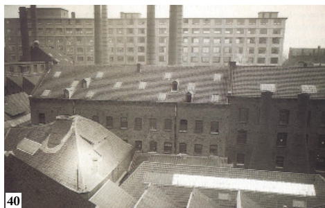
Fig. 40 view towards Eiffel from roof level of extended Brikkenbouw resembling map 1925
