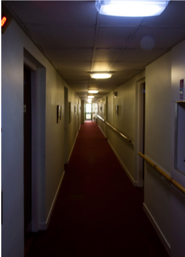
Picture 4.2.6: Corridor with suspended ceiling
