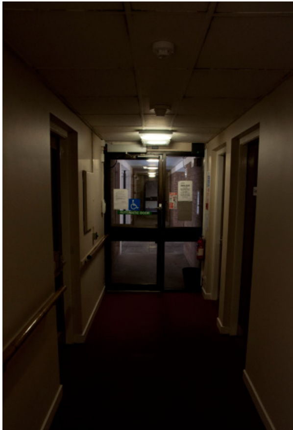
Picture 4.4.2: Back entrance of the building from inside
