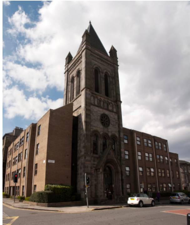
Picture 2.6: Trust Housing Stockbridge (van Niel, 2013)
