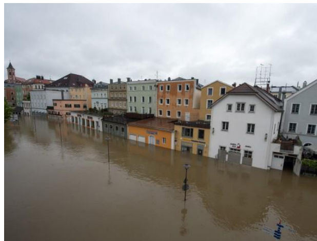
Figure 1.1 Houses in Passau, Germany is flooded because of high water levels of the river Donau. AP / Armin Wiegel www.nrc.nl
