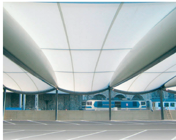
Figure 3.42: Silicone Coated fibreglass for air-supported structures
