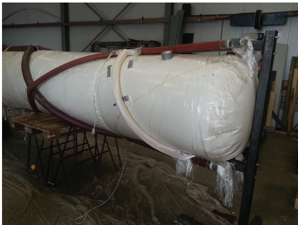
Figure 8.7: fabrication of the crosses
