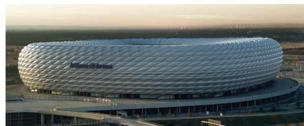
Figure 3.14: The Allianz Arena; the facade is a double membrane structure
