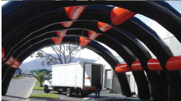
Figure 3.17: TOP; Fuji Pavilion during Expo '70, a discontinuous high pressure system. BOTTOM; Example of a continuous high pressure system.
