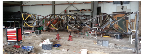
Figure 8.9: Application of the UD carbon/glass layer
