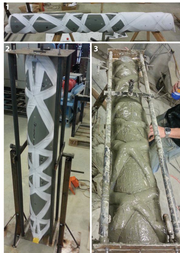
Figure 7.3: 1: Mounting clamps on the PVC piping, 2: Finished mould in the falsework, 3: Casting of the concrete
