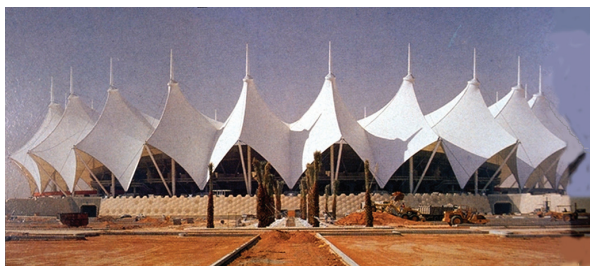
Figure 3.40: PTFE Coated fibreglass on the Riyadh Stadium
