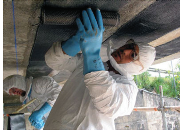
Figure 4.3: Reinforcing an existing concrete bridge with carbon fibres (Freyssinet France)
