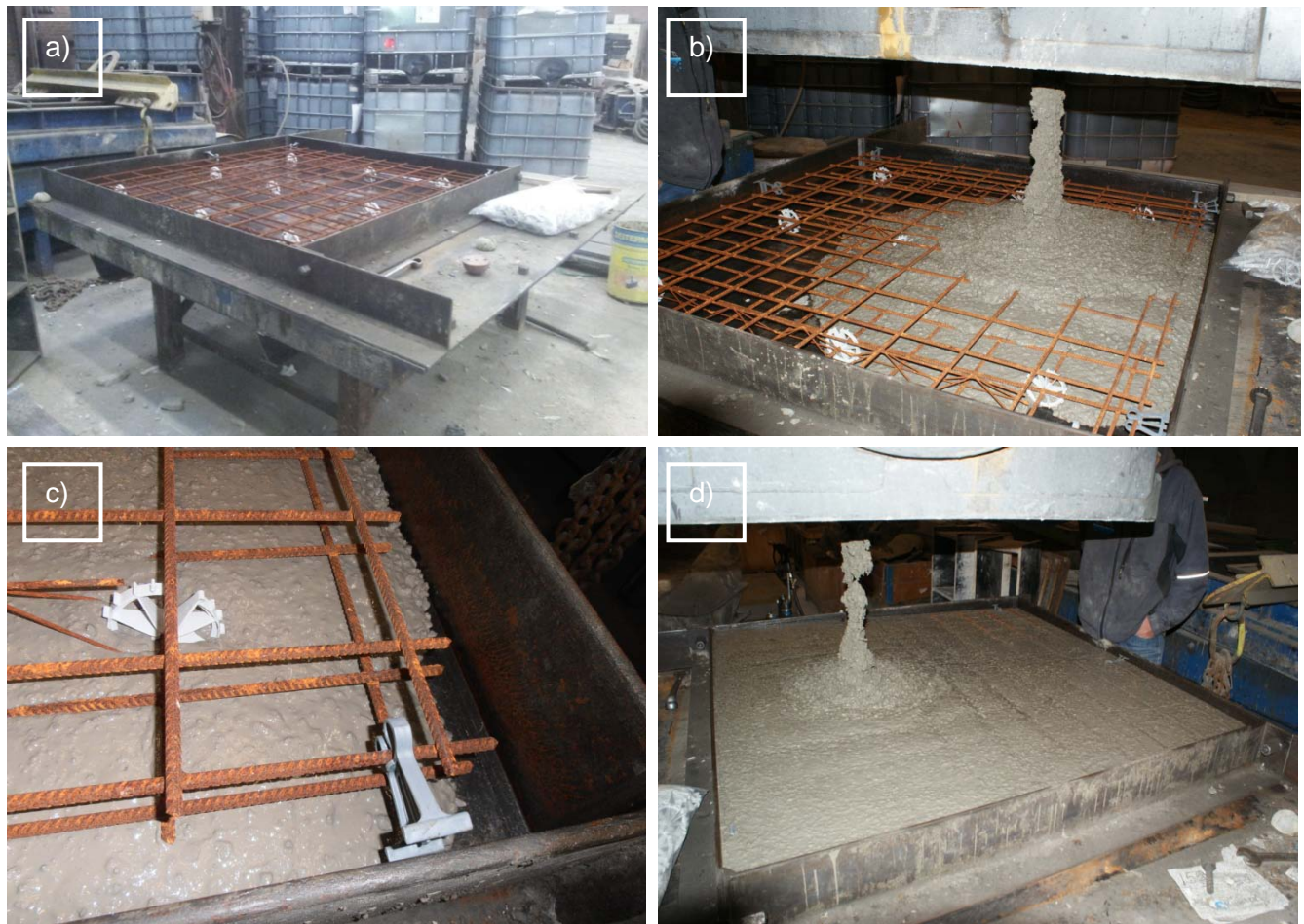
Figure 6-10; SCC real size element a) mold with all reinforcement bars to test blocking in real size b-d) casting the element with SCC batch one, c) filling ability at all corners.
