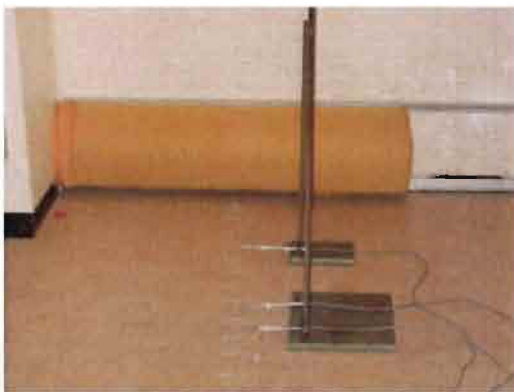
Figure 4.9 Measuring line up with anemometers at several distances from the textile air diffuser
