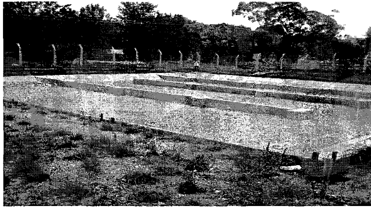
Figure 28 Subsurface Constructed wetland at Kleruu before planting
