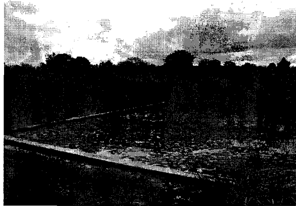
Figure 33 Poorly managed CW at KIBO factory
