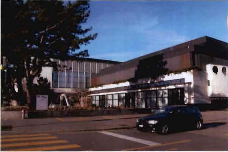
a terrifying brown box instead of the roof terrace
