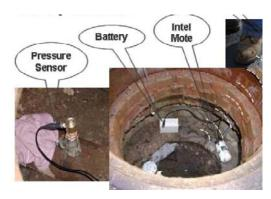
Figure 12: PIPEnet sensor and node (10)
