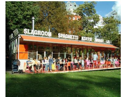
Fig. 4; Teahouse in Breda. The architect John Kormeling subtly plays with our feelings of melancholy. The colors and signs on the roof refer in content and form to the sixties and give the place a warm, familiar feeling.
