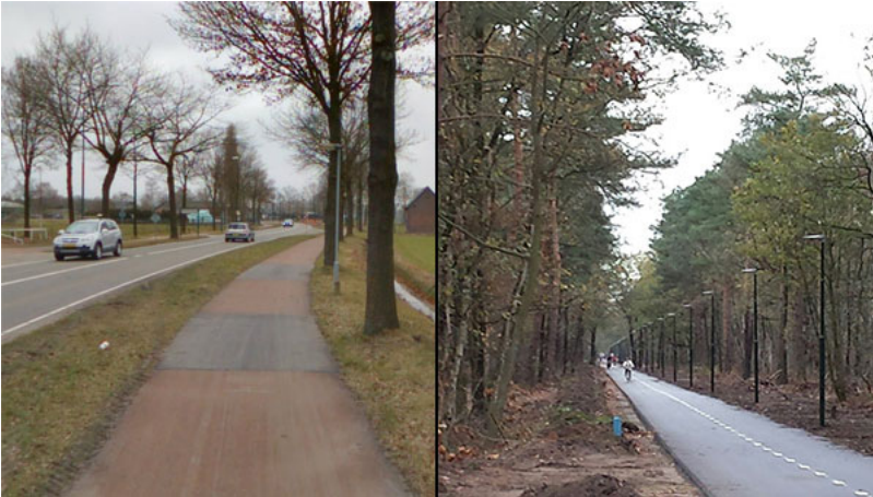
Figure 18: Pavement quality of the route alternative A (left) and alternative B (right)
