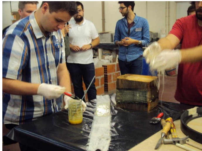
Figure 8: Strengthening techniques, EBR
