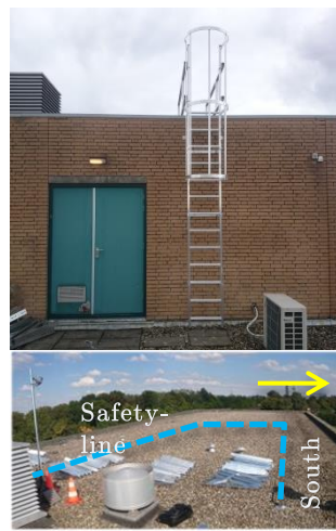
Fig. F.2.6: Safety measures and PV-roof accessibility. New safety stair and fall-off protection with safety line.
