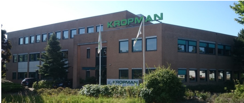
Fig. 4.1: Front view of Kropman Breda office building
