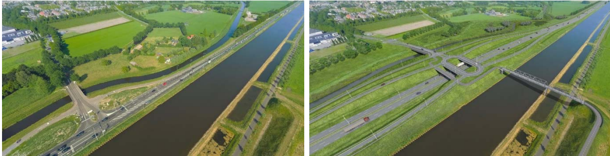
Figure A.0.6. One of the interchanges that is part of the trajectory: the current situation (left) and the design (right)
