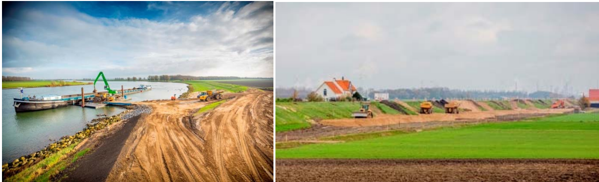
Figure A.0.4. Two images of the project under construction
