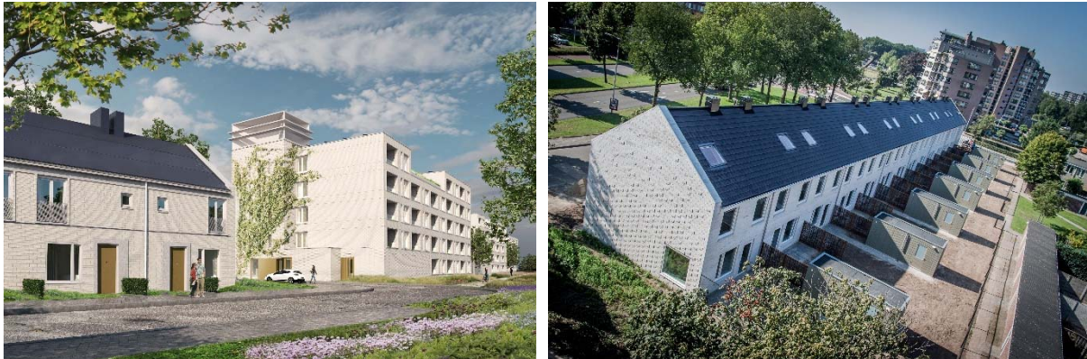
Figure A.0.7. Two render images of the project consisting of apartments and houses
