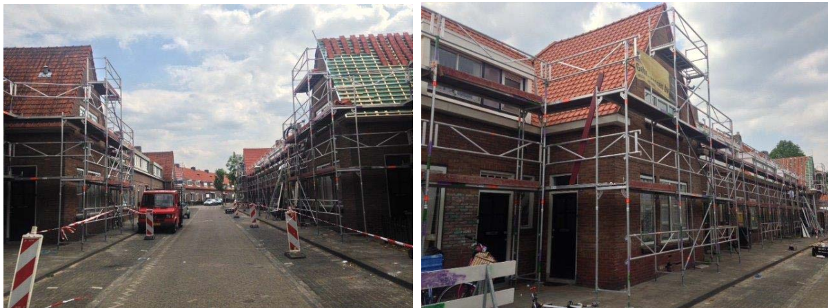
Figure A.0.8. Two photos of the project taken during the renovation
