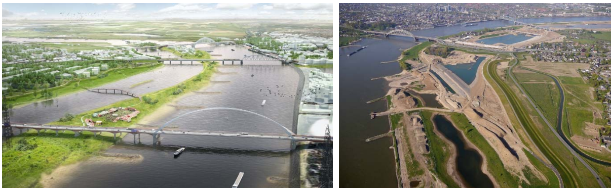
Figure A.0.1. Render image of the project in finished state (left), aerial photo while the largest bridge is extended and traffic led via the bypass (right)
