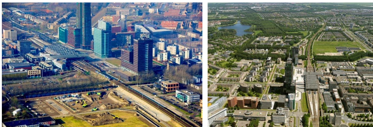
Figure A.0.5. Two aerial photos of the railway trajectory: under construction (left), and before construction (right)
