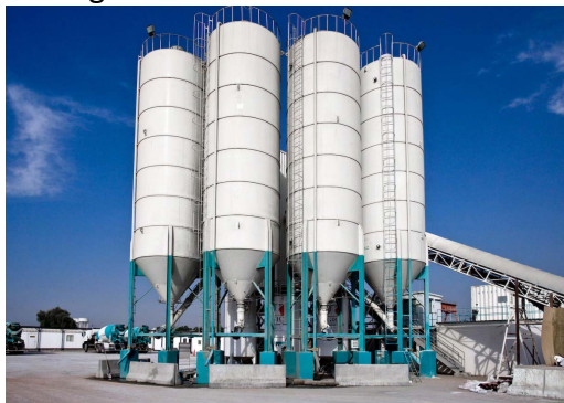
Figure 3.12 Cement production facilities
