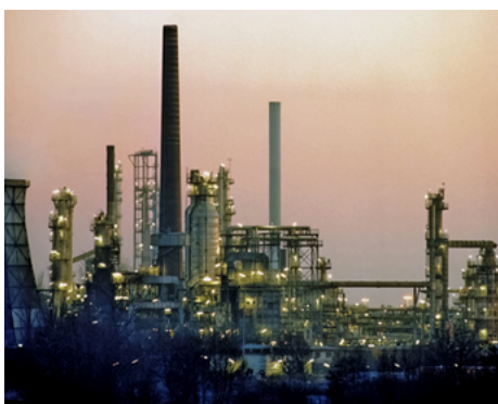
Figure 3.5 Industrial plant with automatic load shedding systems to maintain network stability. Source: Siemens
