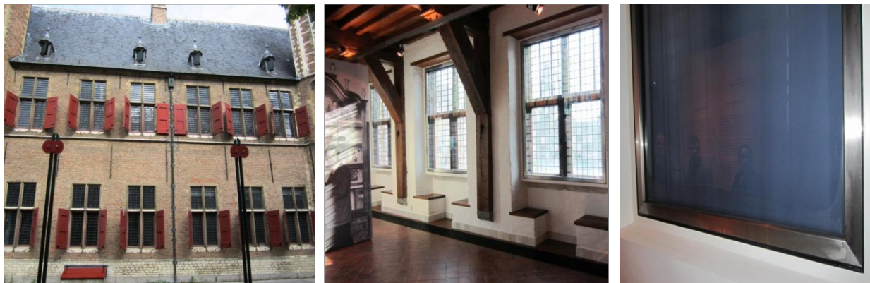
Fig. 5 View of the partial southeastern facade (left) - Picture of the outer wall in exhibition room 2.01 (middle) - Sun screen and additional window (right).
