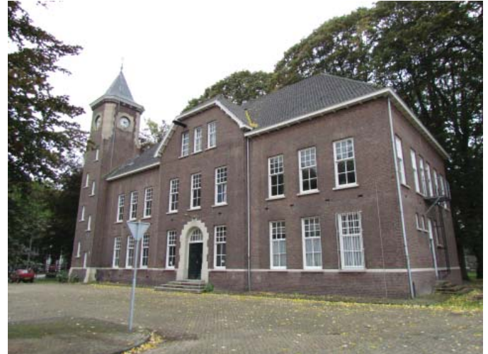
Fig. 20. (above) View from the south-east corner of the terrain, over the Clock Building (the guard building)
