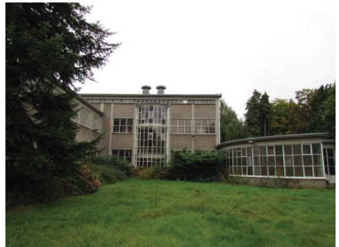
Fig. 24. (below) View of the former hospital building.
