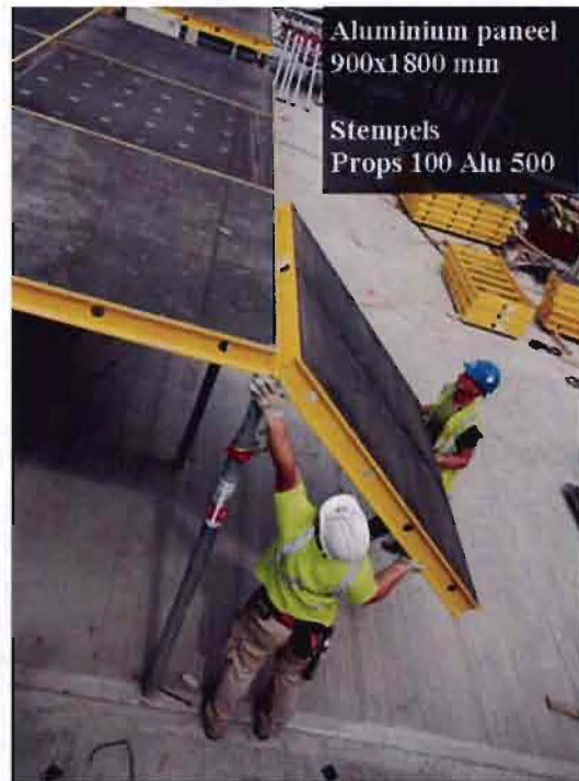
Figuur 41: Principe paneelbekisting
