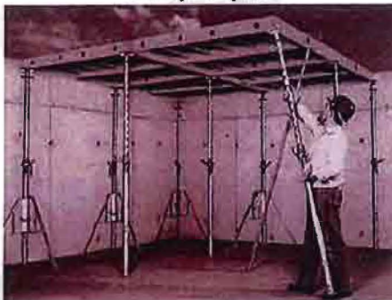
3 Prop the panel
