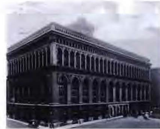
One of the first buildings to use a cage construction which allowed for non bearing outer walls was the Produce Exchange building in New York (1884). Photo: http://www.bc.edu/bc_org/avp/cas/fnart/fa267/19_sky.html
