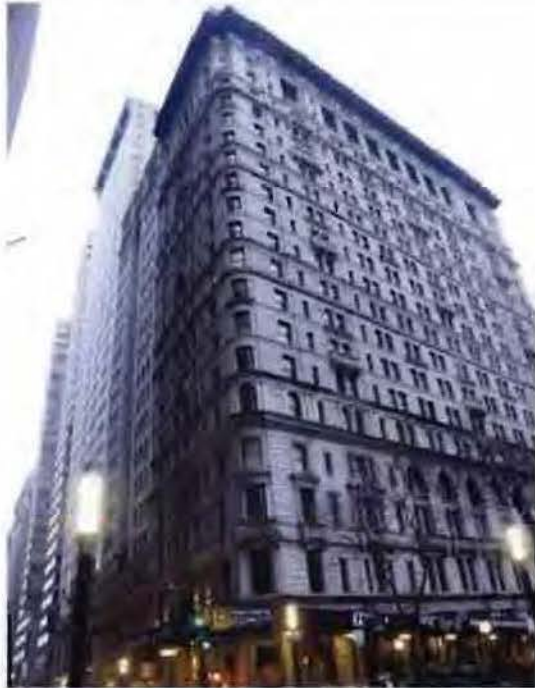
The Empire building in New York (1898). An example of a steel framed building passing the 20 floor mark. Photo: http://en.wikipedia.org/wiki/Empire_Building_(New_York_City)
