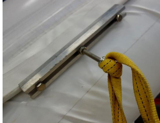
Figure 96: Keder-bolt profile attached on tendon Tensairity arch
