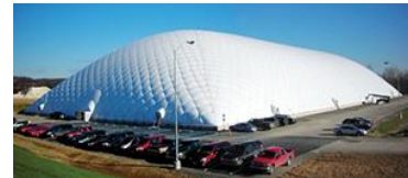
(Big Span structures, N.D.)
