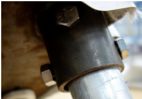
Figure 79: Anchoring of compression element
