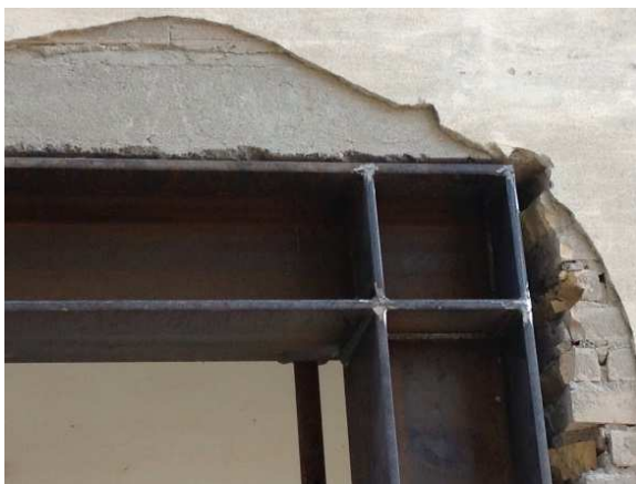
Figure 8-14 Welded Moment Resistant Connection
