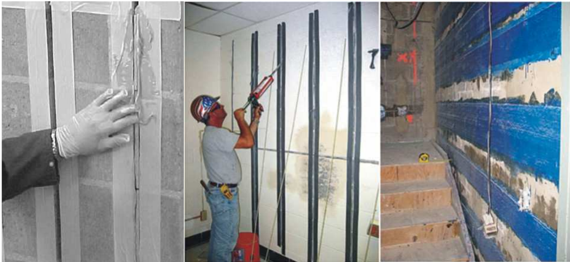
Figure 7-9 URM wall retrofitted using FRP NSM
