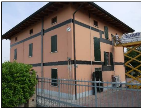
Figure 5-8 Fibre Reinforced Polymers circumferential bandage
