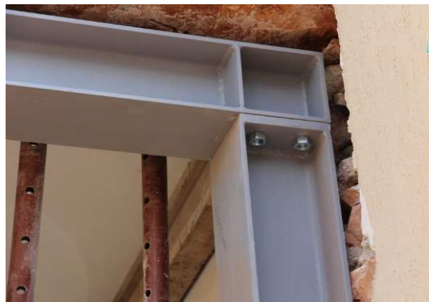
Figure 8-15 Bolted Moment Resistant Connection
