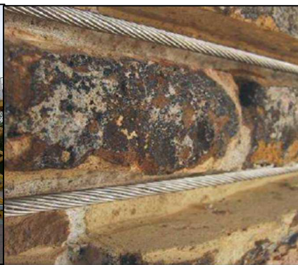
Figure 5-9 Steel ties along the facade
