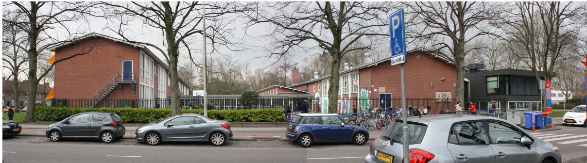
Figure 4.7: View of the school from C
