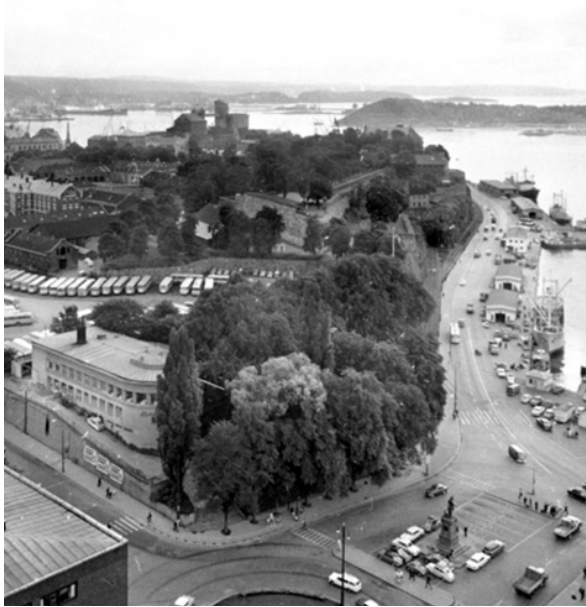
10I Skansen and bus parking in front of Akershus
