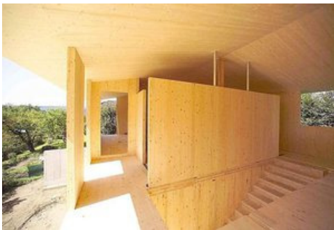
Figure 1.1; CLT structural elements
