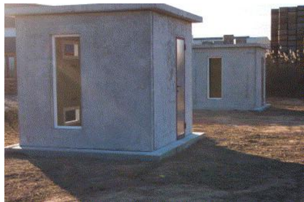
Figure 9: PCM-concrete buildings in Spain.
