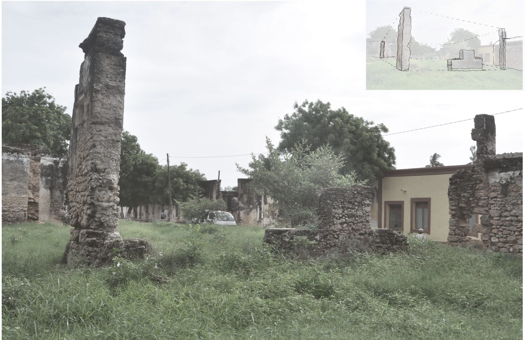
Image 13 - Overview of the volume borders of the former warehouse, 2011-2012
