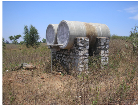
Fig. 5.2: The drinking water tanks of Hanumanthanagara village, these are no longer in use.
