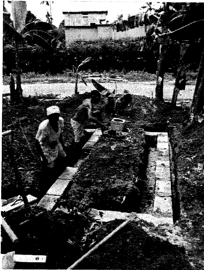
Picture D-6: Laying the foundation (picture taken in Hananasif)
