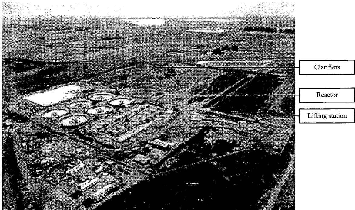
Figure 3: Welgedacht water care works during construction. Picture: ARQ Specialist engineers [45]
