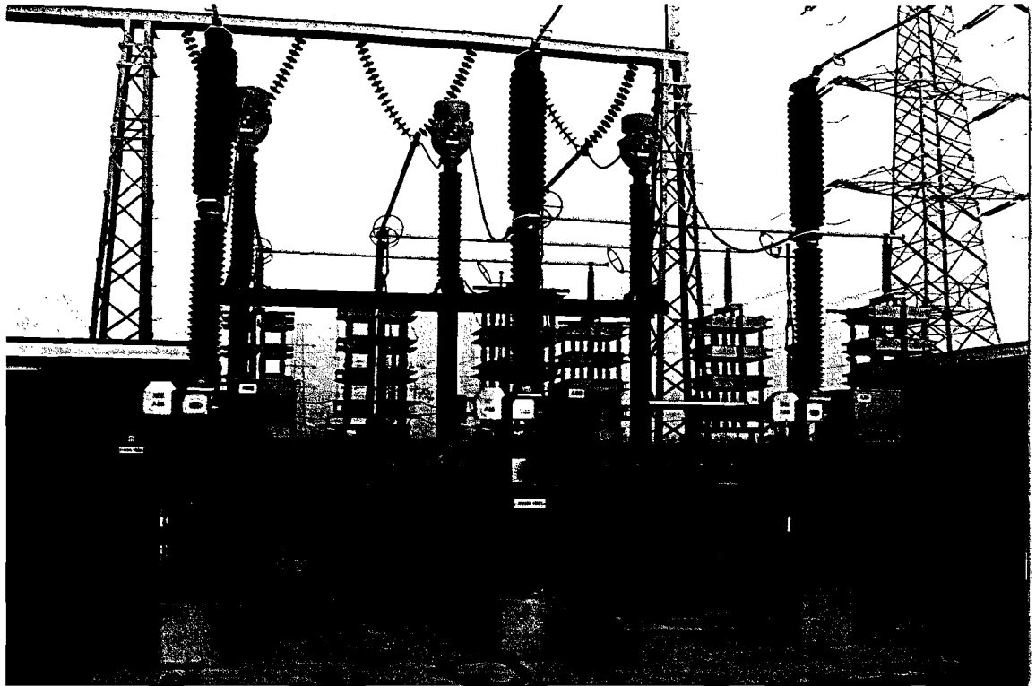
Figure 2 - The ABB (LTB 170 D1) SF 6 Circuit Breaker with Spring Mechanism (BLK52) at Borssele Substation, The Netherlands.
