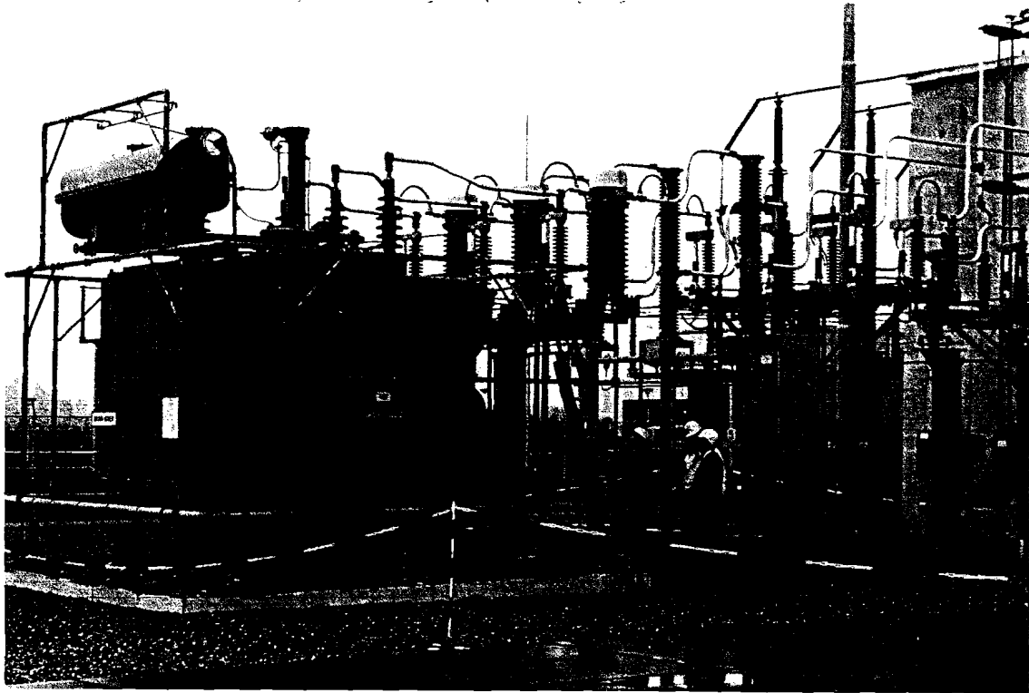
Figure 1 - A 50 MVar tertiary switched shunt reactor at 50 kV. This tertiary reactor is located at Doetinchem Substation, The Netherlands.
