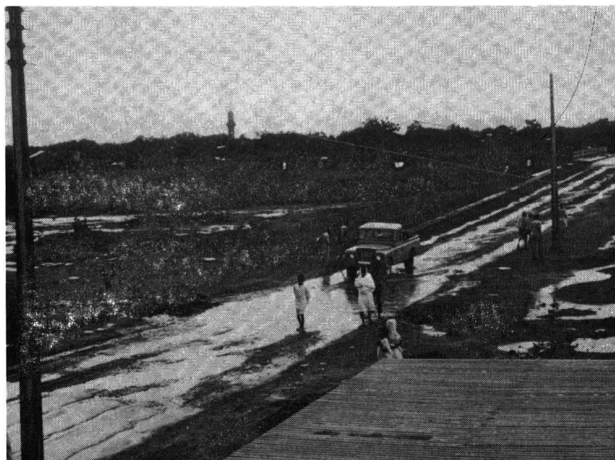
Fig. 5.33 North-West accessroad after short rainfall
