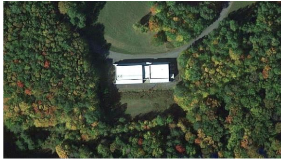
Figure 12. Aerial view of the Celeste Bartos Film Preservation Center
