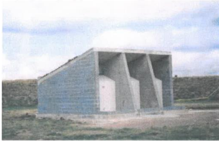
Figure 32. Exterior view of front of facility.
