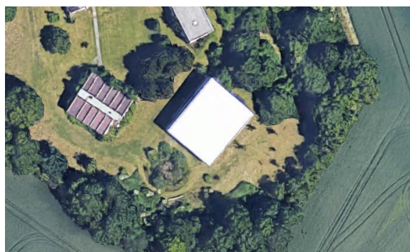
Figure 15. Aerial view of the nitrate vault in Laxenburg
