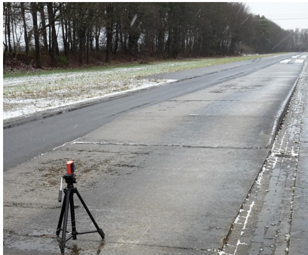
Figure 4.5. Photo of the road bump with laser sensor.
