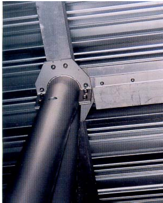
Fig. 55 View of the bolted beam-column connection
