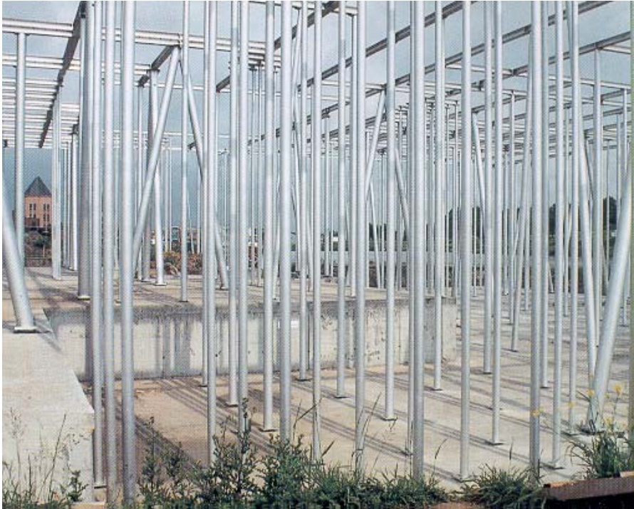
Fig. 54 Floor beams and supporting columns during erection
