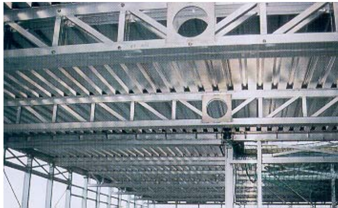
Fig. 57 View of single and double lattice girders
