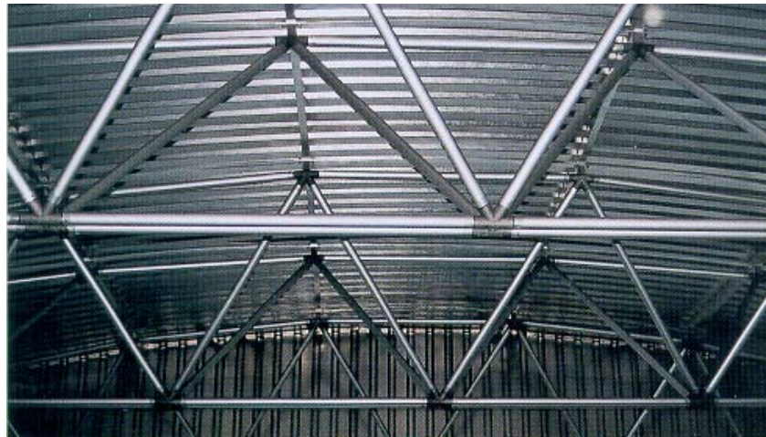
Fig. 60 Triangular truss girders
