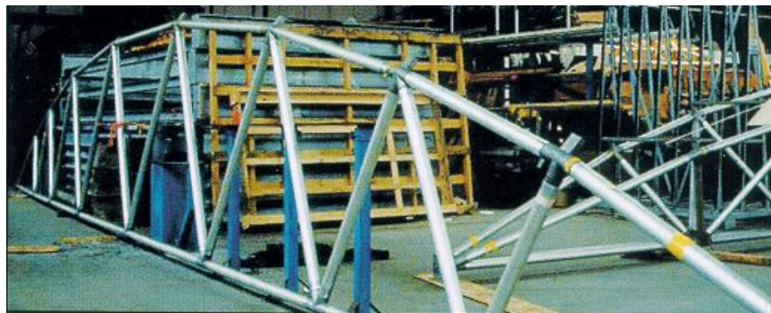
Fig. 61 Shop fabrication of the triangular truss girder
