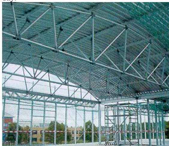
Fig. 64 One day erection at location
