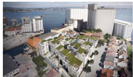
fig. 68 General view, rooftop
