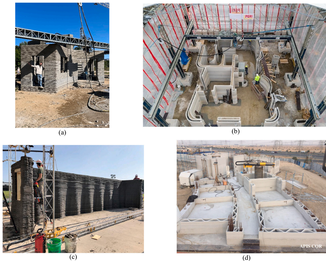
Fig. 6. a–d. On-site printing. (a) Holstebro (credit: COBOD International) and (b) Beckum Houses, both with a larger-than-building BOD2 printer, on one position. (c) B-Hut with a gantry on 2 subsequent positions. (d) Dubai office with cylindrical robot, on 12 positions.
