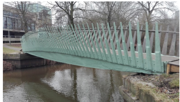
Fig. 3: Bio-based bridge at Eindhoven University of Technology campus
