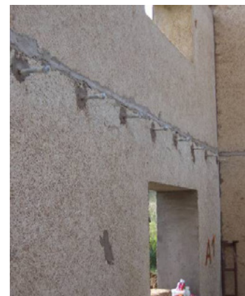
Figure 24 - Anchors in ring beam for floor support
