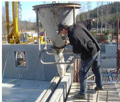
Figure 23 - Pouring of concrete
