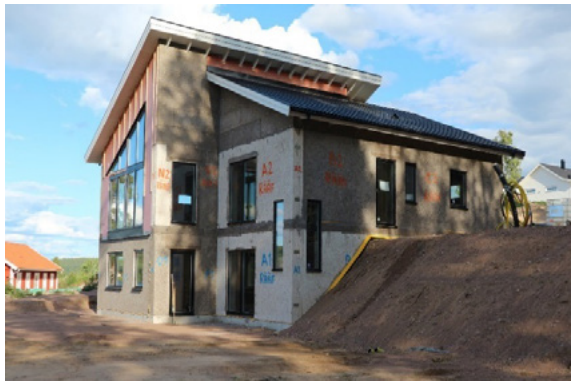
Figures 25, 26 - two-story villa under construction (Träullit, Sweden)
