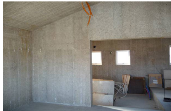
Figure 10 - WSCB Plant with EltoBoard Press Figure 11 - WSCB applied in walls, floors and roof (Takemura, Japan)
