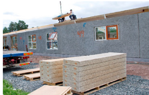
Figure 4 - Reinforced Roofing Boards
