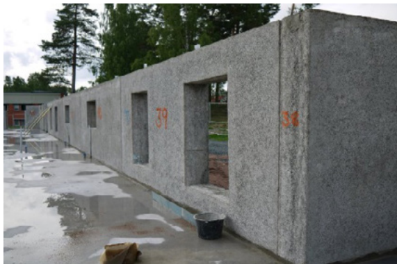
Figures 25, 26 - two-story villa under construction (Träullit, Sweden)
