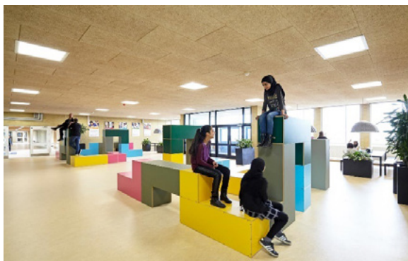
Figure 3 - Acoustic ceiling panels in public building
