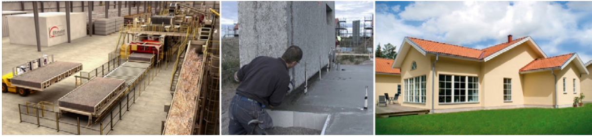
Figure 16 – Collage of Large Element System: Production, Installation and a Finished Large Element House.
