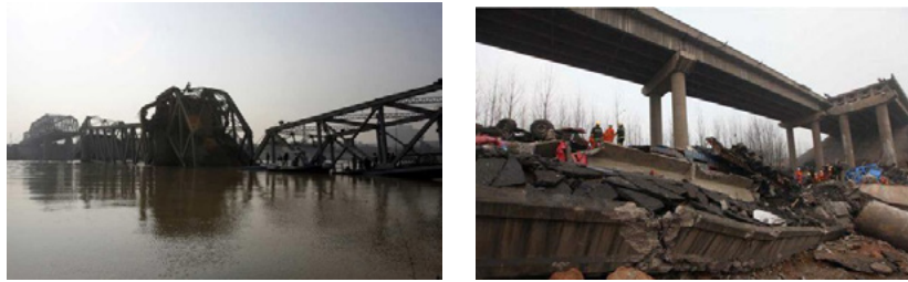
1a) The collapsed Sarafiya Bridge 1b) The collapsed Yichang Bridge
