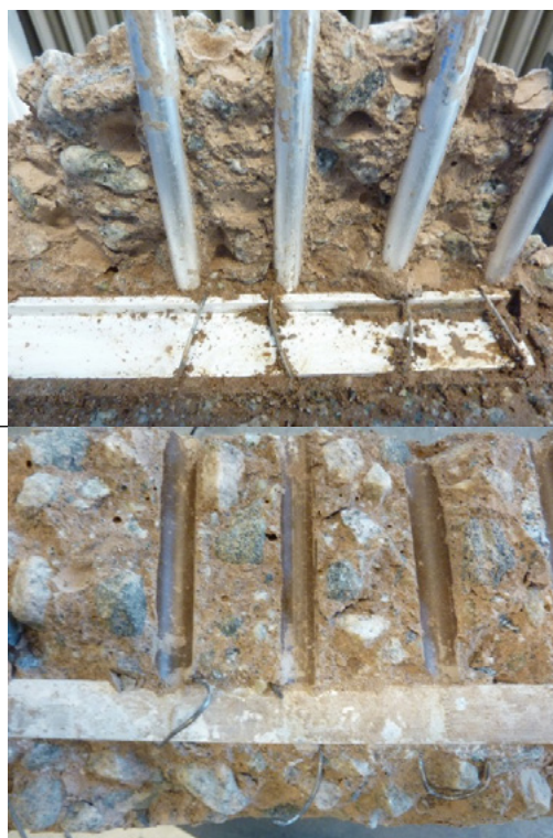
Figure 3: Aluminium alloy round bars and T-bar (top) of beam after chiselling it open and their imprints (bottom) showing no signs of corrosion products after 40 days moist curing at 20°C.
