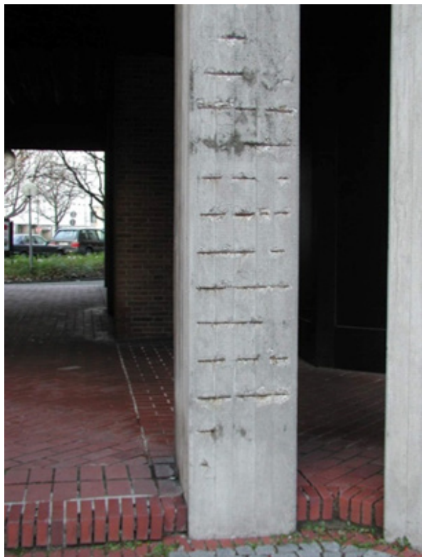
Figure 5: Reinforced concrete pillar, photo Gehlen
