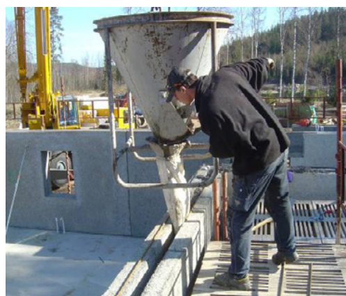
Figure 22 - Open Ring-beam Figure 23 - Pouring of concrete
