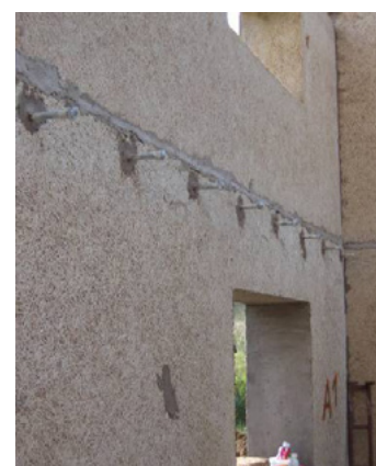
Figure 24 - Anchors in ring beam for floor support
