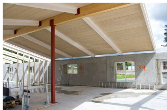
Figures 27, 28, 29, 30 – Construction of a highly insulated day-care centre in Sweden, utilising Large Elements for the outer walls and Reinforced Roofing Boards for the roof (Träullit, Sweden)
