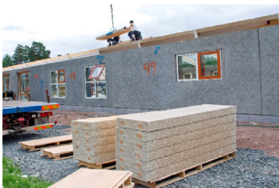
Figures 27, 28, 29, 30 – Construction of a highly insulated day-care centre in Sweden, utilising Large Elements for the outer walls and Reinforced Roofing Boards for the roof (Träullit, Sweden)
