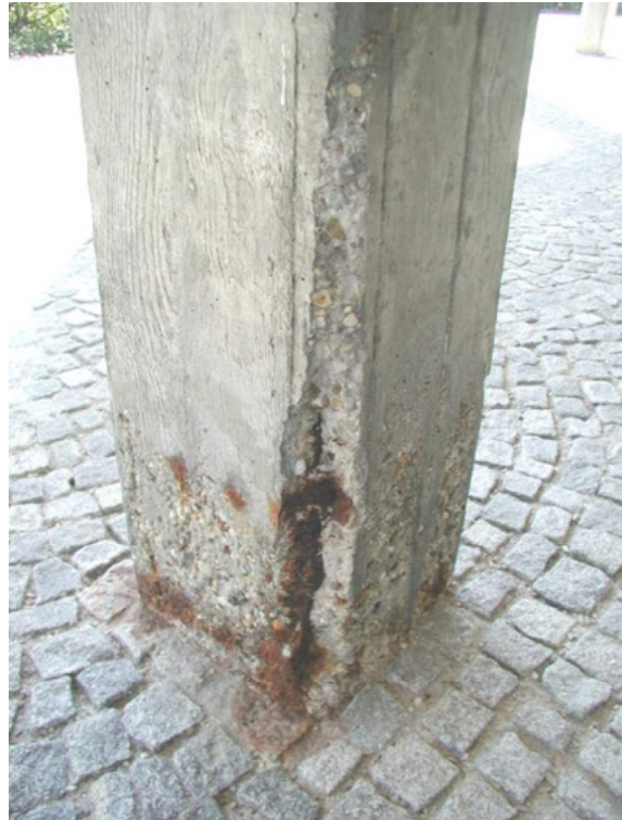
Figure 1: Mechanically loaded concrete column, affected by chloride in de-icing salts which has induced corrosion of rebar and freeze-thaw scaling, photo Gehlen
