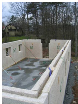
Figure 22 - Open Ring-beam Figure 23 - Pouring of concrete
