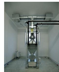
► Fig. 4: View of inside of a cell with existing HVAC system
