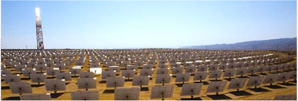
Fig. 54: Solar tower plant (Brightsource Energy, 2011)
