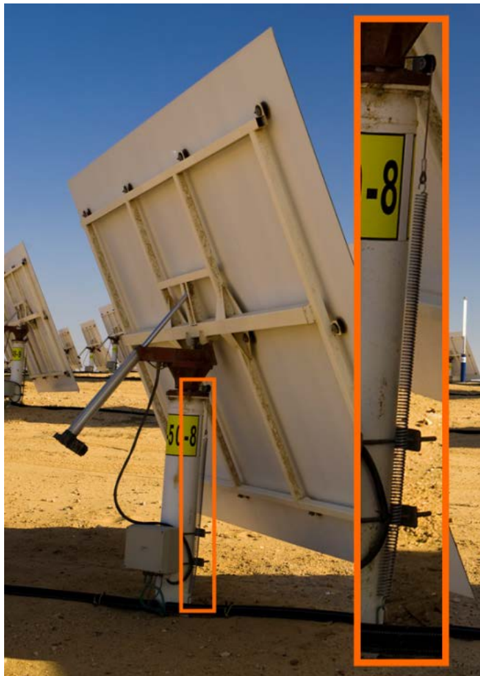
Fig. 3: Heliostat with pre-tensioned azimuth drive via spring (Brightsource Energy, 2012)
